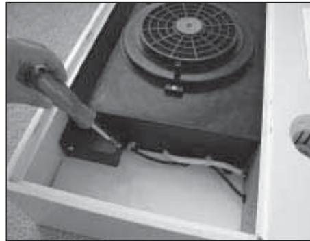
2. Remove cover from junction box to gain access to electrical wiring.
